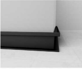
⑥ Installation finished
